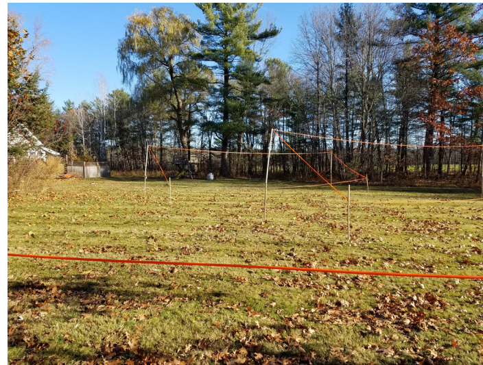
Grading sticks of various lengths are used to simulate the pitch of the array
