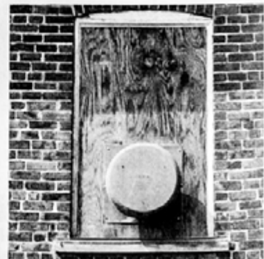
c. The exhaust fan has tamper-proof housing.
