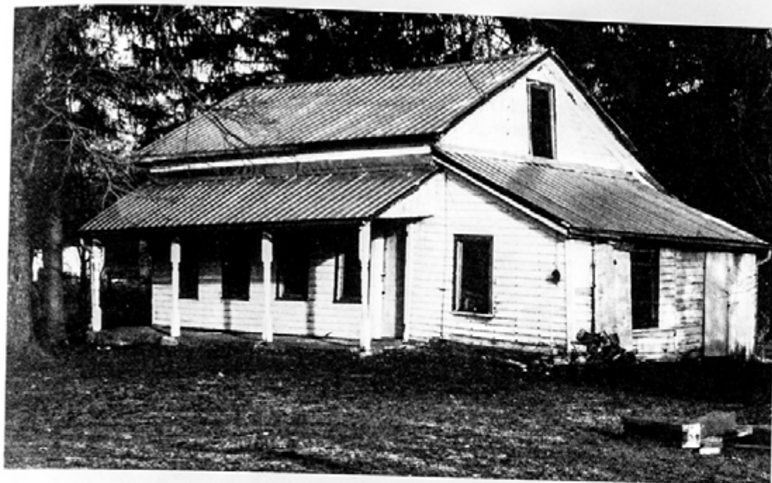
Figure 7. Non-historic materials are appropriate for mothballing projects when they are used to protect historic evidence remaining for future preservation. This lightweight aluminum channel frame and roofing covers the historic wooden shingle roof. Galvanized mesh panels secure the window openings from intrusion by raccoons and other unwanted guests. Photo: Williamsport Preservation Training Center, NPS.
