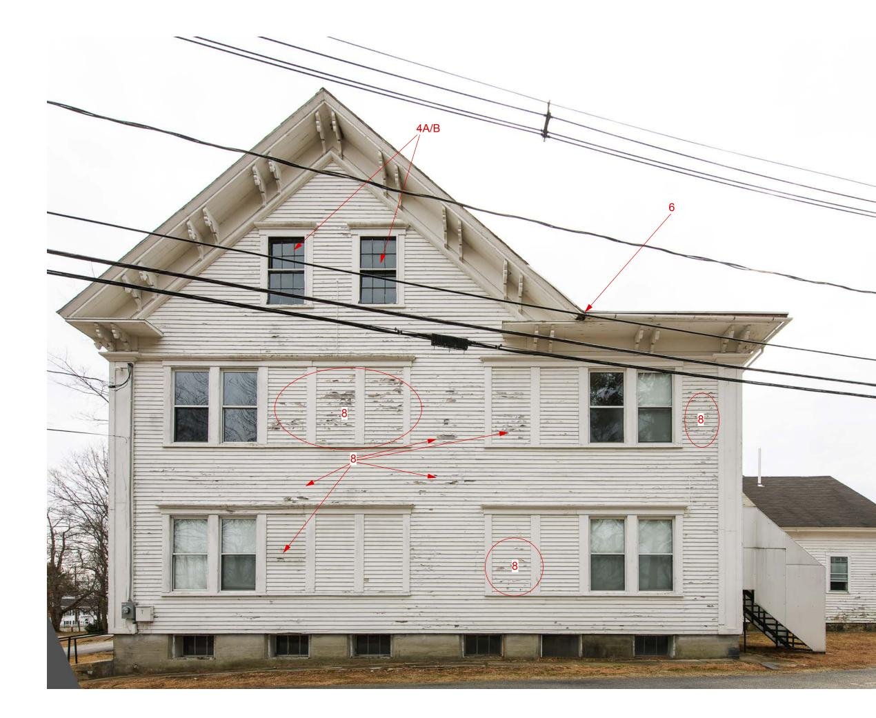
4A/B. NORTH ELEVATION GABLE WINDOWS NOT PROTECTED BY STORM WINDOWS, LOWER SASH RIGHT WINDOW APPEARS TO TILT INWARDS, (SEE DETAIL IMAGES). STABILIZATION RECOMMENDATION: INSTALL STORM SASH. 6. JOINT AT INTERSECTION OF
