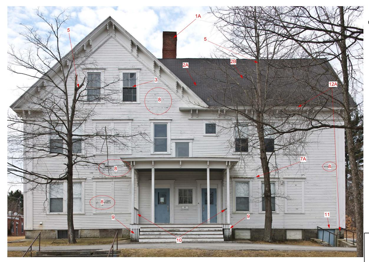
1A. CHIMNEY, MISSING MASONRY UNITS, CRACKING, MORTAR JOINT DETERIORATION, (SEE DETAIL IMAGE). NOTE: MOST DAMAGE OCCURS ABOVE LOWER DRIP/BELT COURSE.
