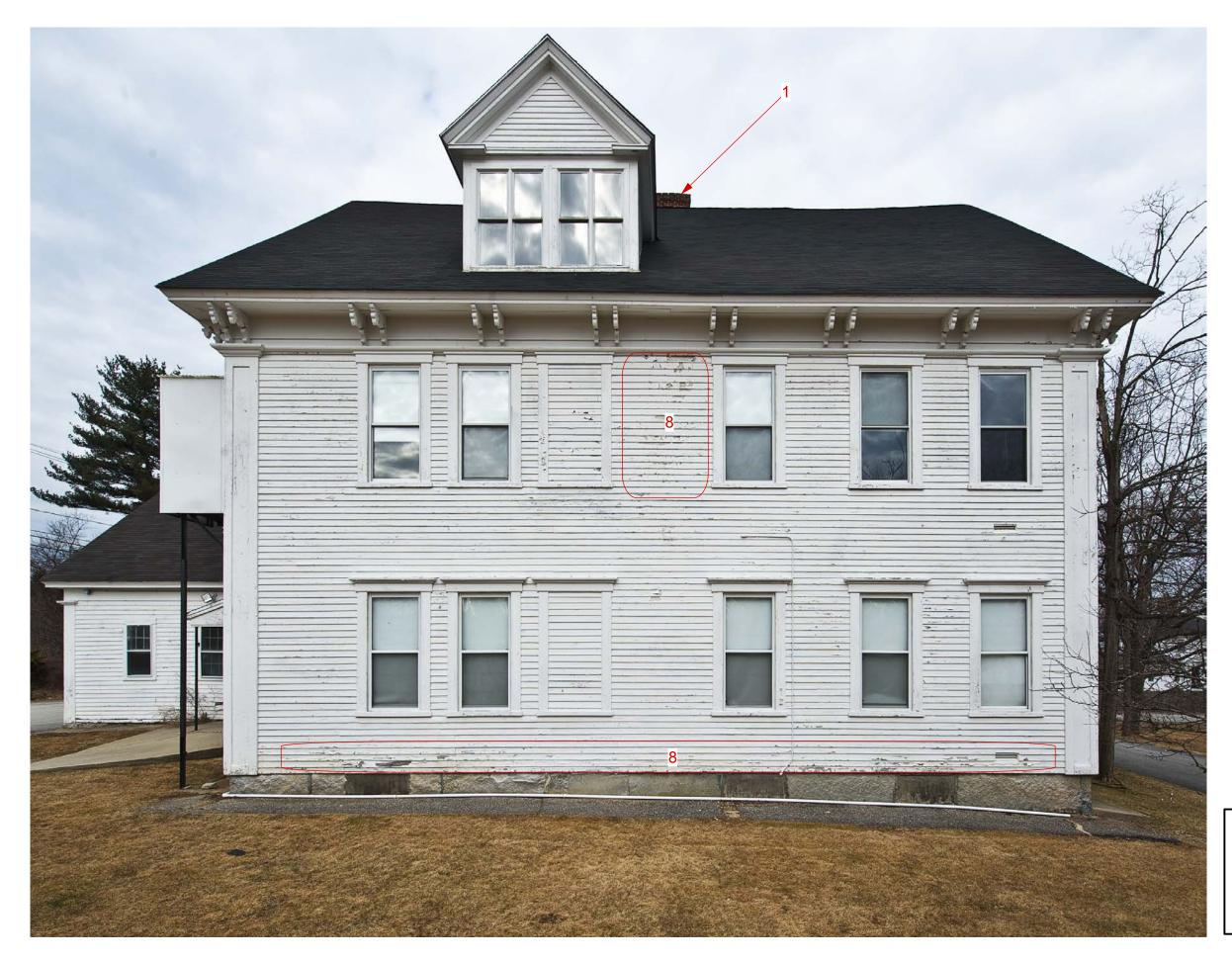
1. SOUTH FACE OF CHIMNEY, MISSING MASONRY UNITS, CRACKING, MORTAR JOINT DETERIORATION, (SEE DETAIL IMAGES). NOTE: MOST
