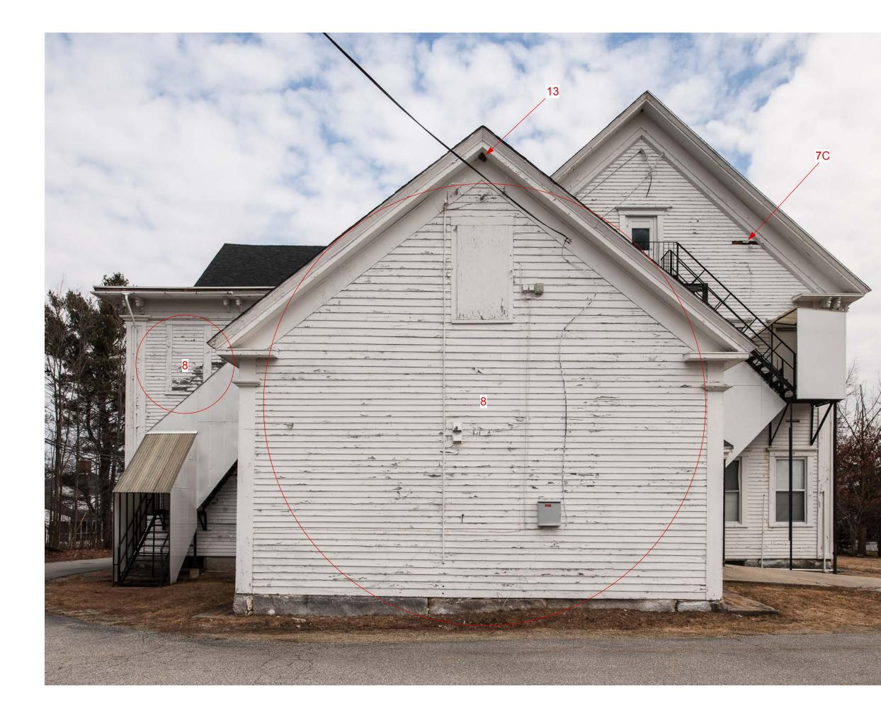
7C. DAMAGED/MISSING CLAPBOARD, (SEE DETAIL IMAGE). STABILIZATION RECOMMENDATION: REPLACE/REPAIR CLAPBOARD. 8. SIGNIFICANT AREAS OF PAINT LOSS/FAILURE ON BOTH THE EAST & NORTH ELEVATIONS, IN MANY CASES PAINT FAILURE HAS EXPOSED THE WOOD SUBSTRATE. STABILIZATION RECOMMENDATION: PAINT PRIME AREAS OF BARE WOOD WITH OIL BASED PRIMER. 13. BEE/WASP/HORNET NEST. STABILIZATION RECOMMENDATION: REMOVE NEST.
