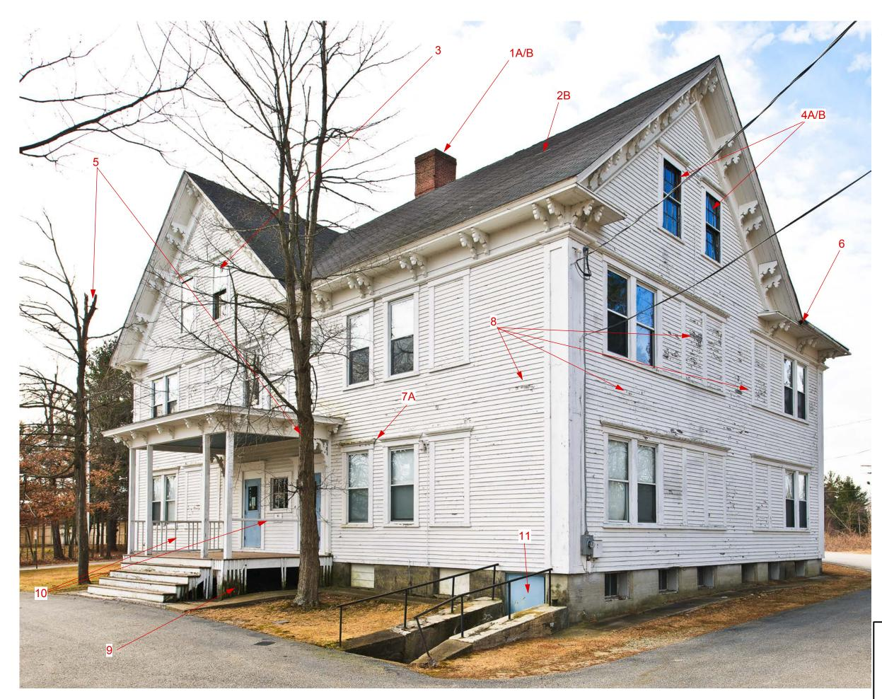
1A/B. CHIMNEY, MISSING MASONRY UNITS, CRACKING, MORTAR JOINT DETERIORATION, (SEE DETAIL IMAGES). NOTE: MOST DAMAGE OCCURS ABOVE LOWER DRIP/BELT COURSE.
