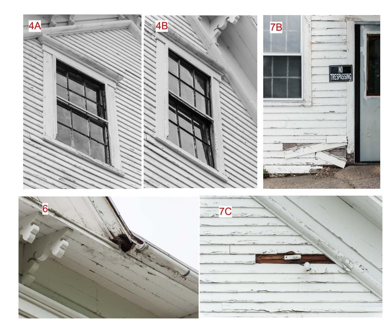
4A/B. NORTH ELEVATION GABLE WINDOWS NOT PROTECTED BY STORM WINDOWS, LOWER SASH RIGHT WINDOW (4B) APPEARS TO TILT INWARDS. STABILIZATION RECOMMENDATION: INSTALL STORM SASH. 6. NORTH ELEVATION, JOINT AT INTERSECTION OF RAKING & LEVEL FASCIA BOARDS IS OPEN TO THE INTERIOR OF THE ROOF FRAMING & MORE THAN LARGE ENOUGH TO
