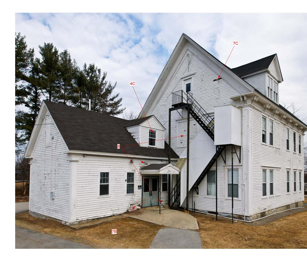
4C. SOUTH ELEVATION DORMER WINDOW HAS NO STORM WINDOW. STABILIZATION RECOMMENDATION: INSTALL STORM WINDOW. 7B/C. DAMAGED/MISSING CLAPBOARD, (SEE DETAIL IMAGES). STABILIZATION RECOMMENDATION: REPLACE/REPAIR CLAPBOARD. 8. SIGNIFICANT AREAS OF PAINT LOSS/FAILURE ON BOTH THE EAST & NORTH ELEVATIONS, IN MANY CASES PAINT FAILURE HAS EXPOSED THE WOOD SUBSTRATE. STABILIZATION RECOMMENDATION: PAINT PRIME AREAS OF BARE WOOD WITH OIL BASED PRIMER.
