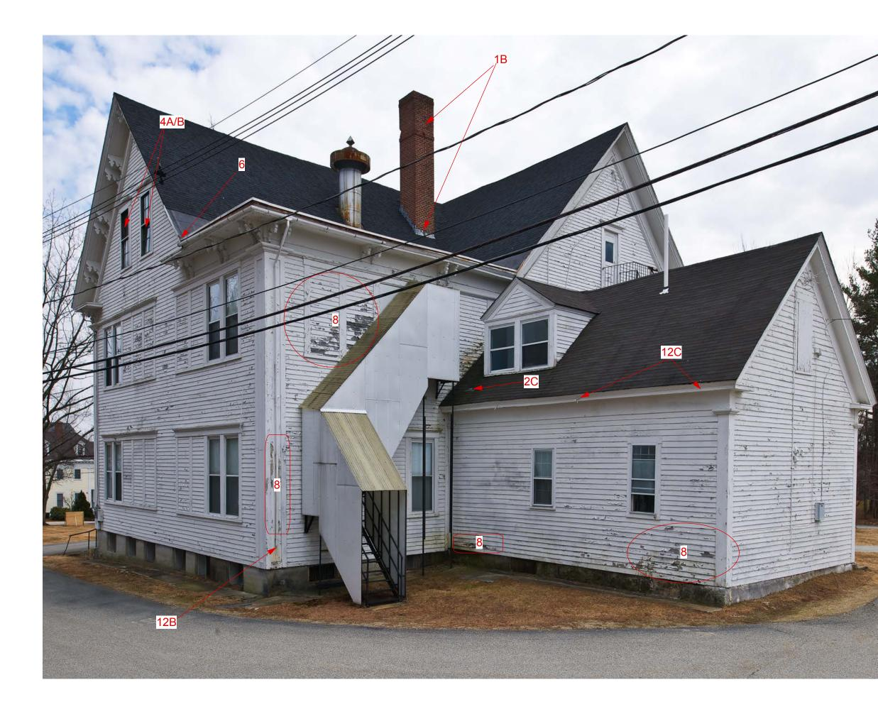
1B. NORTH & WEST FACES OF CHIMNEY, MISSING MASONRY UNITS, CRACKING, MORTAR JOINT DETERIORATION, (SEE DETAIL IMAGES). NOTE: MOST DAMAGE OCCURS ABOVE LOWER DRIP/BELT COURSE. CHIMNEY STACK FLASHING/COUNTER FLASHING NEEDS INSPECTION.
