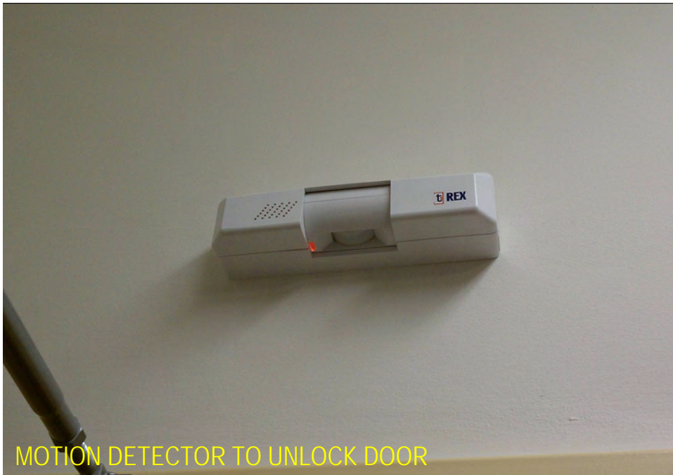
MOTION DETECTOR TO UNLOCK DOOR
