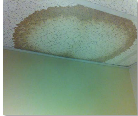
Figure 4: Water Stain from Roof Leak
