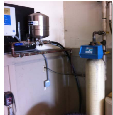
Figure 14: Domestic Water Treatment System
