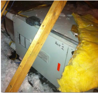
Figure 19: Attic Air Handling Unit
