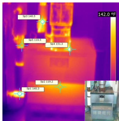
Figure 24: Peerless Boiler IR
