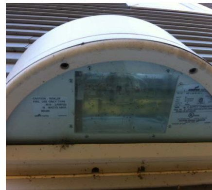
Figure 12: Exterior MH Fixtures
