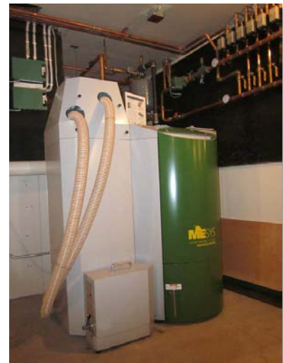
Figure 25: Automated Wood Pellet Boiler (Maine Energy Systems®)
