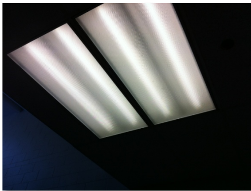
Figure 15: T8 Light Fixtures in Vestibule
