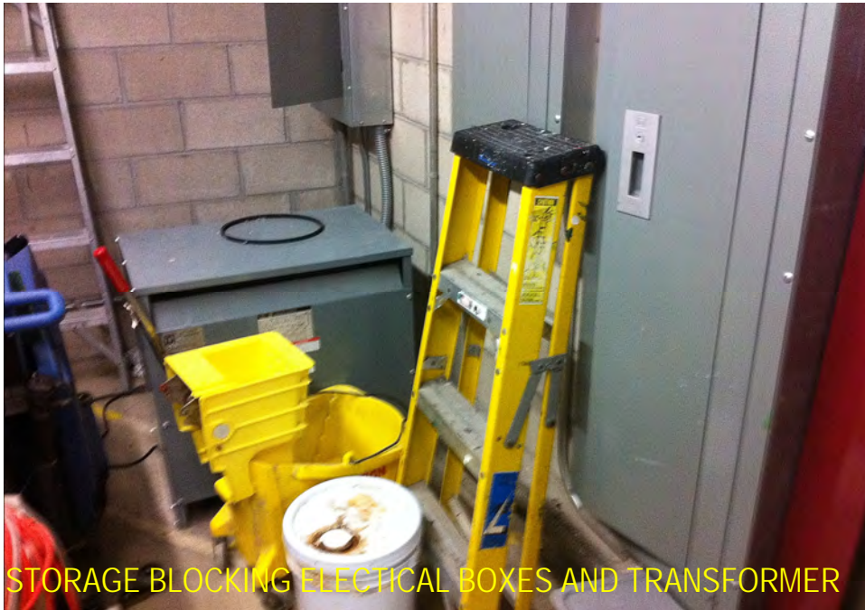
STORAGE BLOCKING ELECTRICAL BOXES AND TRANSFORMER
