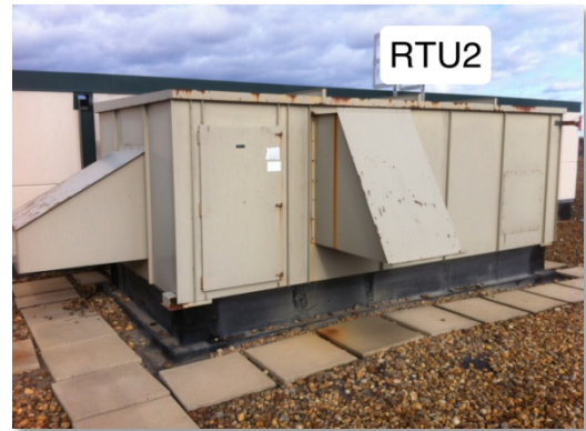
Figure 21: Rooftop AHU
