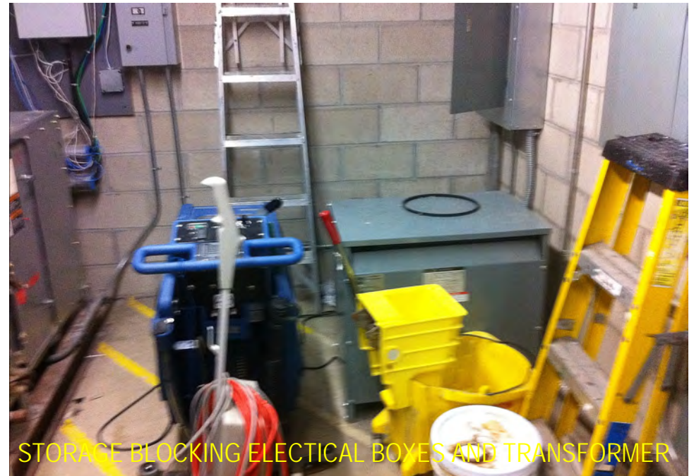
STORAGE BLOCKING ELECTRICAL BOXES AND TRANSFORMER
