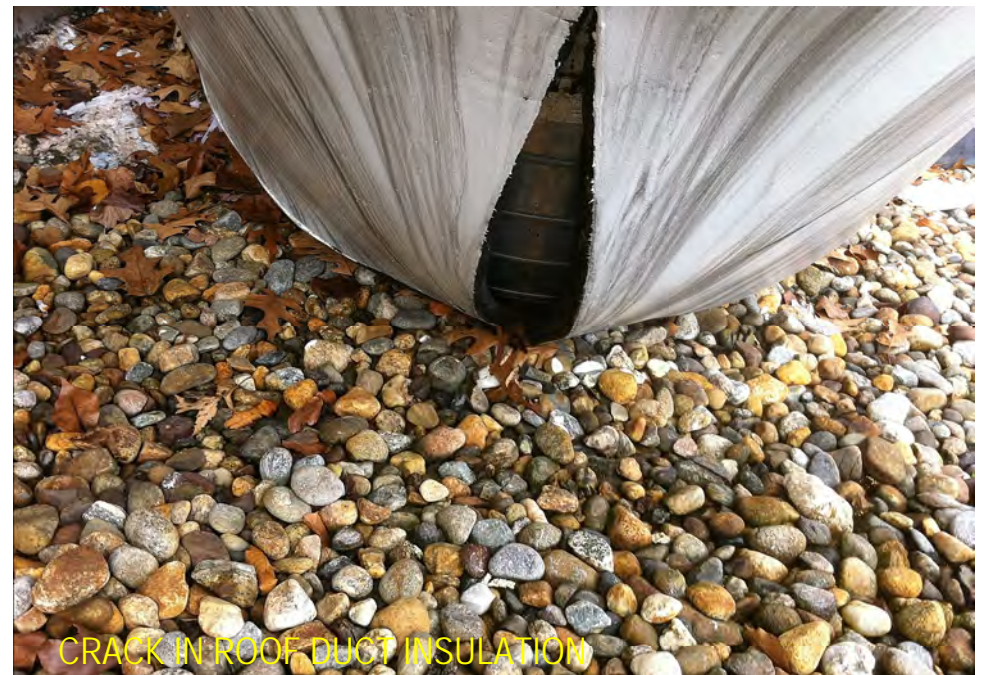
CRACK IN ROOF DUCT INSULATION
