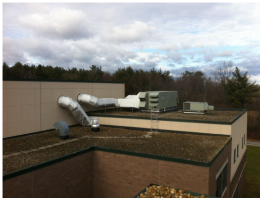
Figure 9: Multi-Level Ballasted Roof
