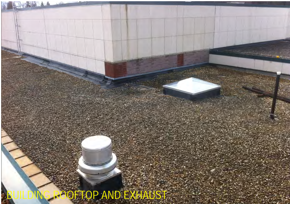
RUSTED AND CRACKED EXHAUST ON ROOFTOP
