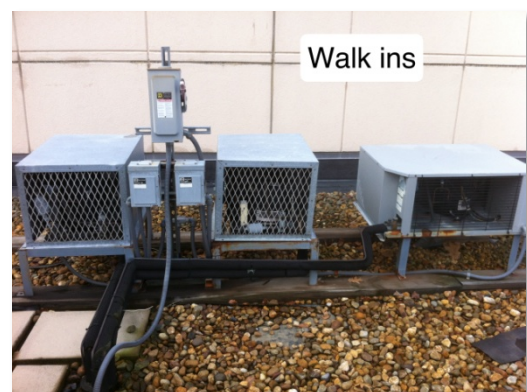
Figure 20: Walk-in Freezer Condensers on Roof
