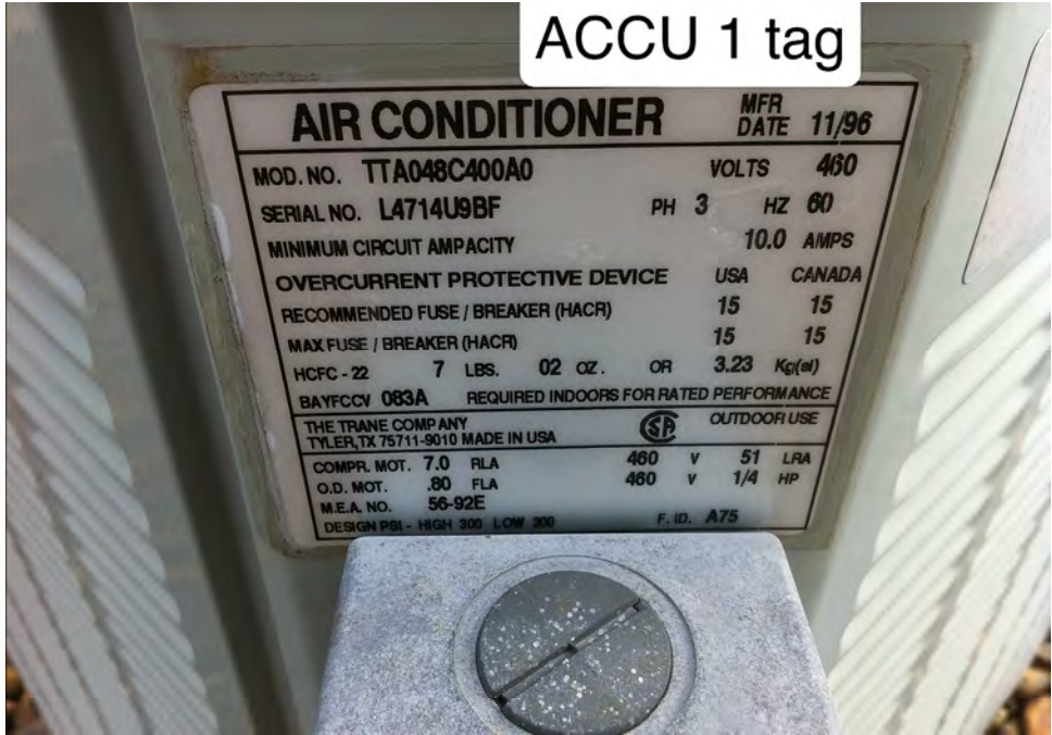
ROOFTOP AIR CONDITIONER CONDENSING UNIT ACCU1
