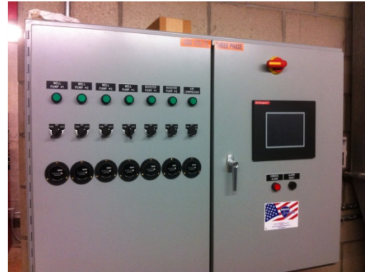
Figure 17: Well Pump Controllers in Boiler Room
