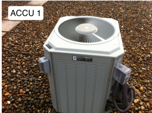
Figure 19: Air Condition Condensing Unit 1 on Roof Modern cooling systems can achieve SEERs up to 24. As example, replacing a unit with a SEER rating of 8 with a new unit rated at 16 would reduce energy consumption by 50% and provide an equivalent cooling capacity.
