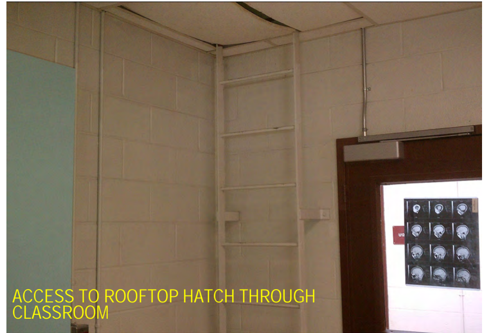
UNUSED HATCH WAS CLOSED BUT NOT SEALED. RECOMMEND SEALING HATCH TO REVENT THERMAL TRANSFER.
