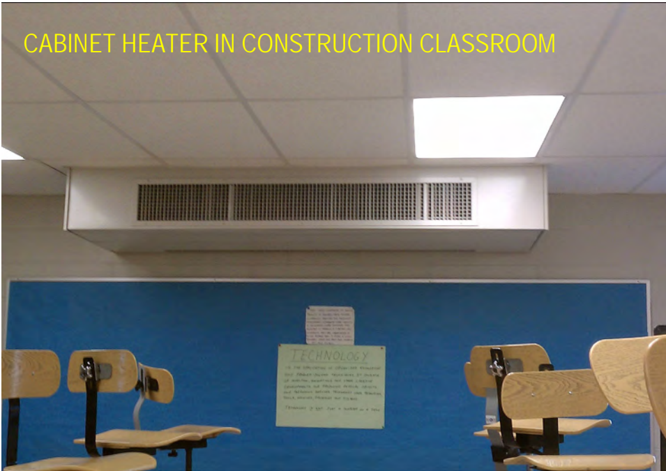
UNIT HEATER IN CONSTRUCTION WORKROOM. RECOMMEND SEALING THROUGH WALL PENETRATIONS
