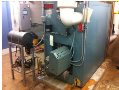
Figure 18: Hot Water Boiler
