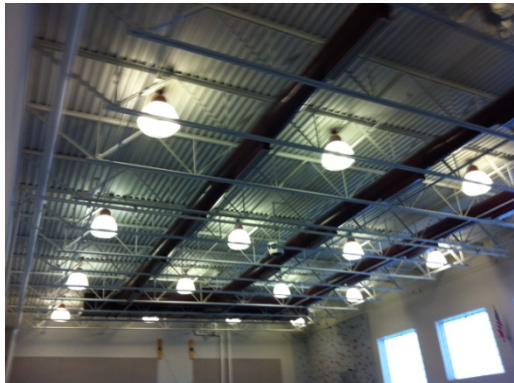
Figure 15: High Wattage CFL Fixtures in Multi-Purpose Room
