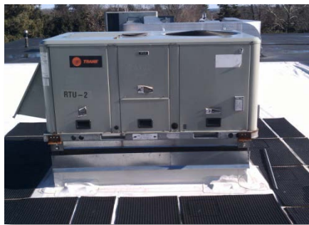
Figure 21: Rooftop Unit 2 Ventilation
