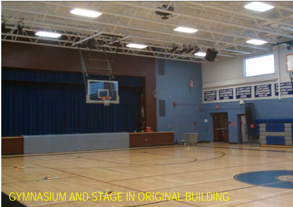
T8 LIGHT FIXTURE WITH 6 BULBS IN GYMNASIUM
