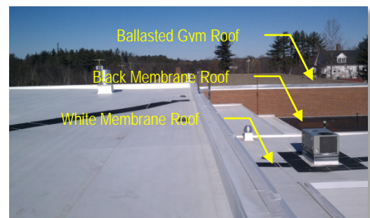
Figure 10: Multi-Level Membrane Roof
