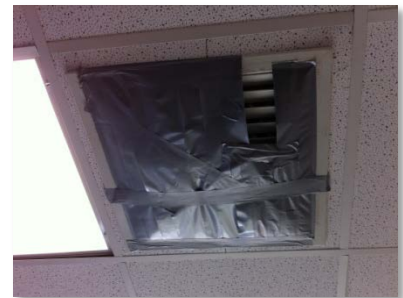
Figure 5: Blocked Vent in Room 144
