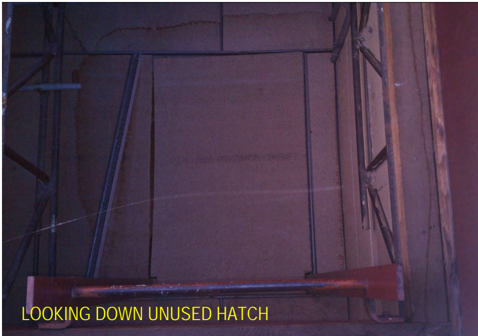
UNUSED HATCH WAS CLOSED BUT NOT SEALED. RECOMMEND SEALING HATCH TO REVENT THERMAL TRANSFER.
