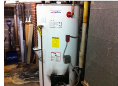
Figure 17: Domestic Hot Water Heater
