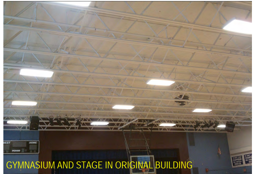
T8 LIGHT FIXTURE WITH 6 BULBS IN GYMNASIUM
