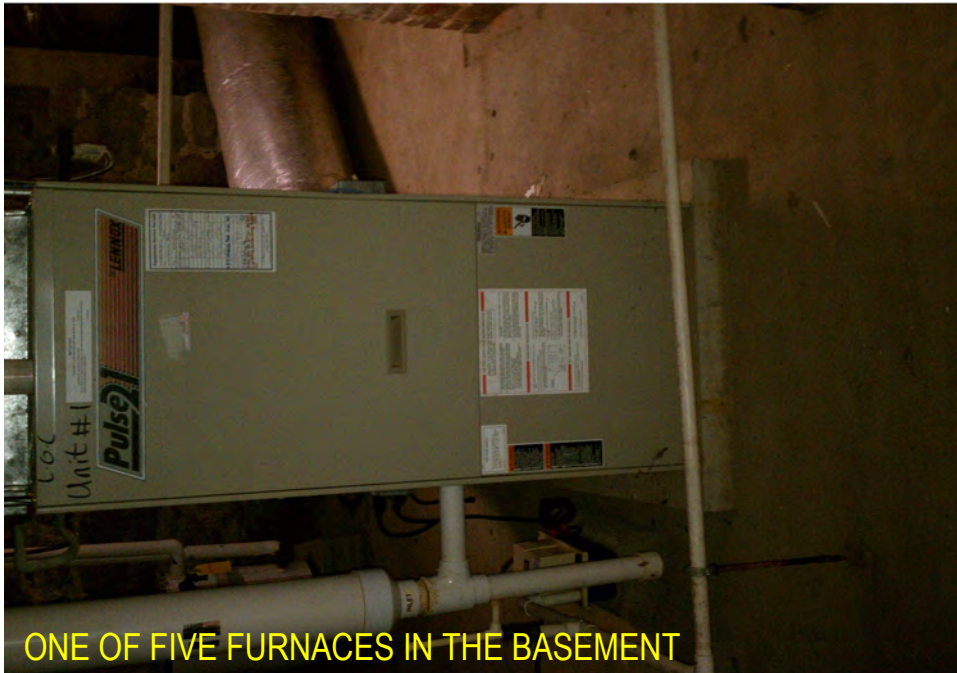
FURNACE ELECTRICAL BOX AND CONDENSATE DRIP LINE
