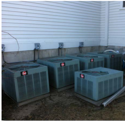
Figure 20: Rheem® Condensers
