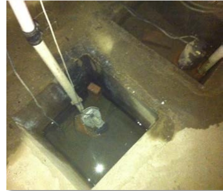
Figure 5: Basement Sump Pumps
