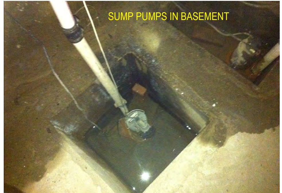
SUMP PUMPS IN BASEMENT
