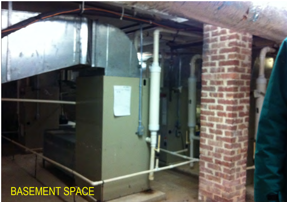
ONE OF FIVE FURNACES IN THE BASEMENT
