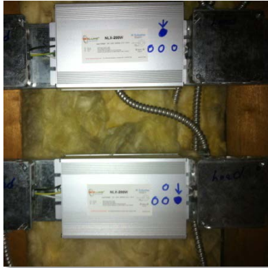
Figure 14: Induction Light Ballasts
