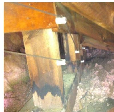
Figure 13: Knob and Tube Wiring in 1910 Attic
