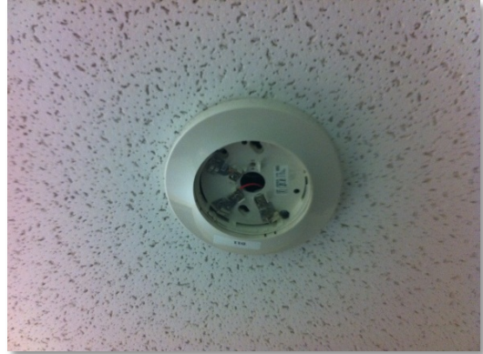
Figure 15: Removed smoke detection device
