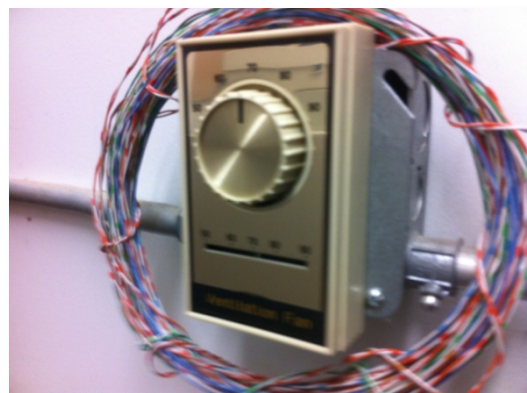
Figure 13: Radio Room Exhaust Ventilation Fan Controls
