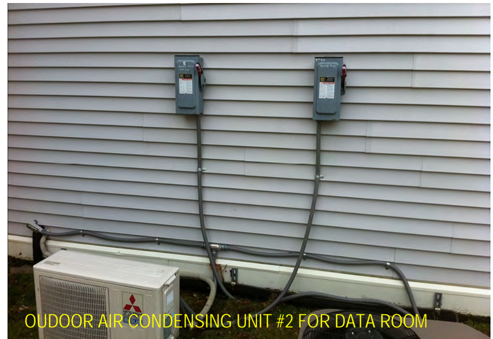
ELECTRICAL DISCONNECT FOR DATA ROOM UNIT
