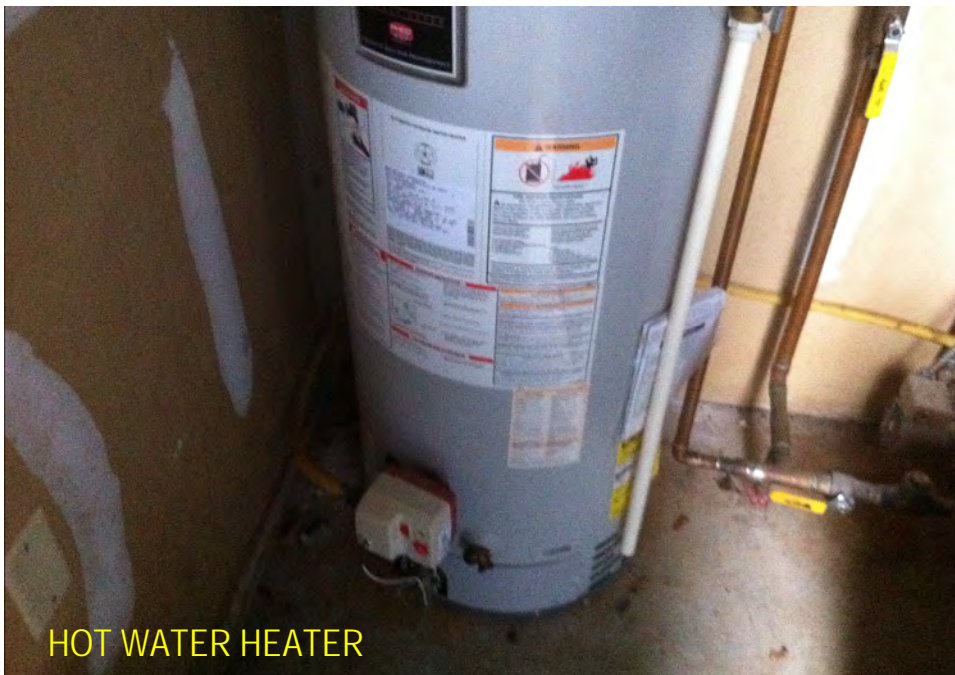
UNINSULATED HOT WATER PIPES ALLOW THERMAL LOSS
