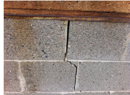
Figure 19: Crack in Chimney Blocking
