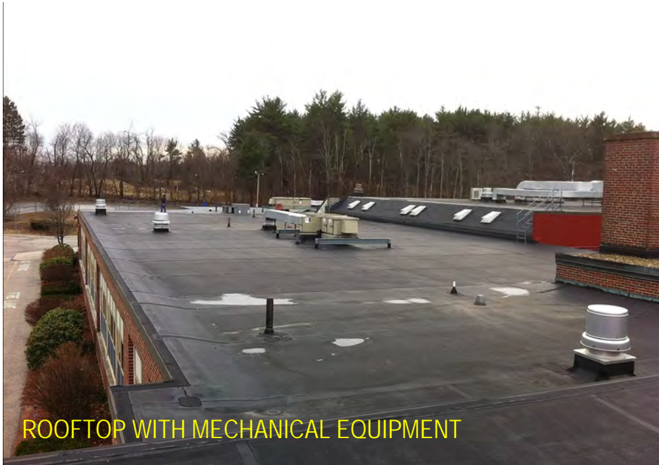
ROOFTOP AIR HANDLING UNIT FOR LIBRARY
