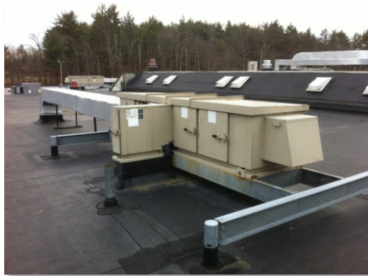
Figure 15: Packaged Rooftop AHU (typ.)
