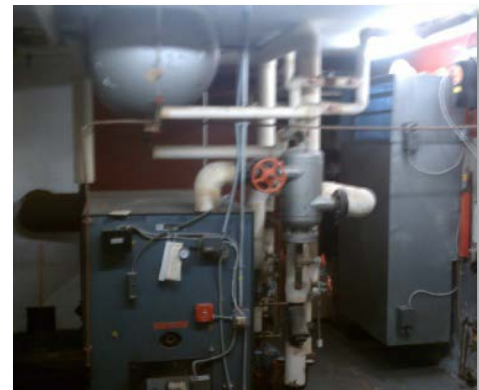
Figure 14: 1 of 2 Boiler Rooms with 1 of 2 Weil McLain Boilers
