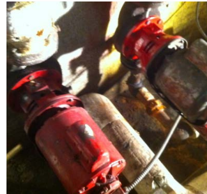
Figure 16: Circulating Pumps in Boiler Room #1
