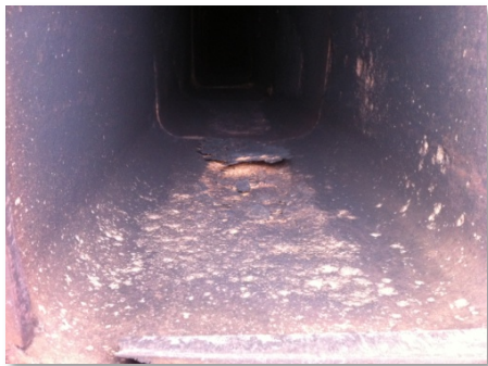
Figure 18: Deteriorating Flue (note spalling section)
