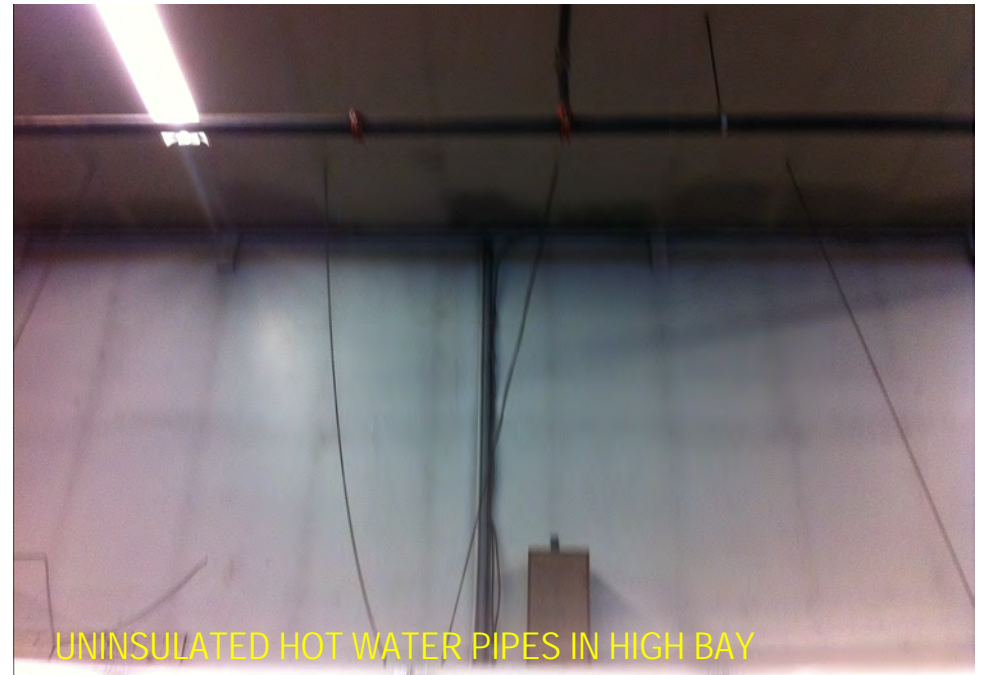
UNINSULATED HOT WATER PIPES IN HIGH BAY
