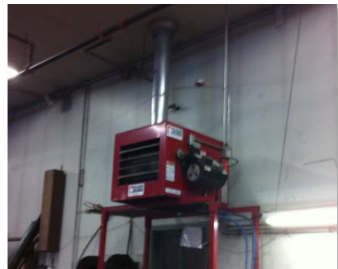
Figure 12: Waste Oil Furnace
