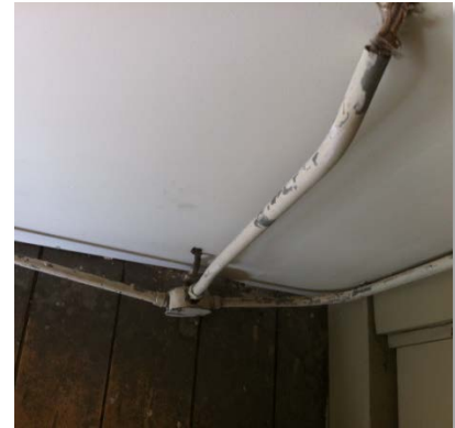
Figure 13: Exposed Electrical Wiring
