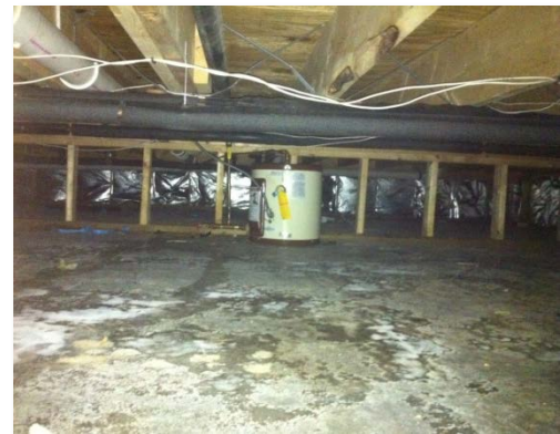
Figure 17: DHW Tank in Addition Crawlspace
