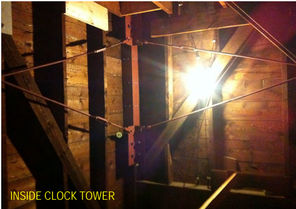
SUPPORT BRACING IN CLOCK TOWER
