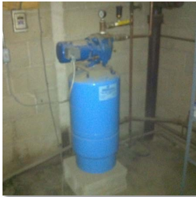
Figure 15: Water Booster Pump
