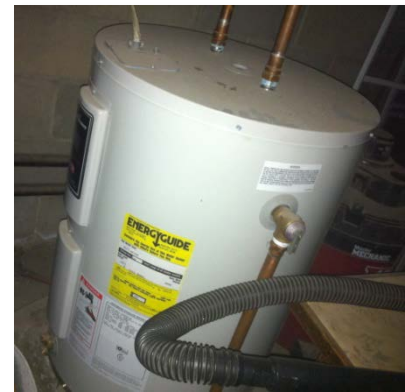
Figure 16: Main DHW Tank
