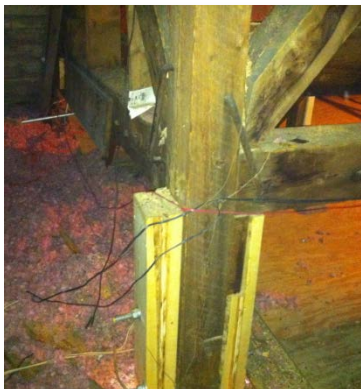
Figure 9: Attic Insulation, Reinforced Beam, Exposed Wiring
