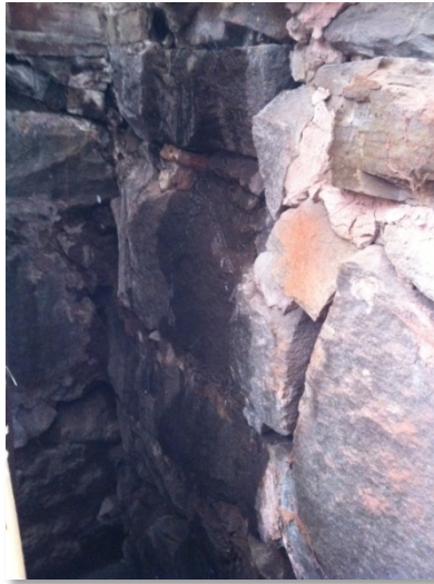
Figure 21: Seepage through Basement Wall
