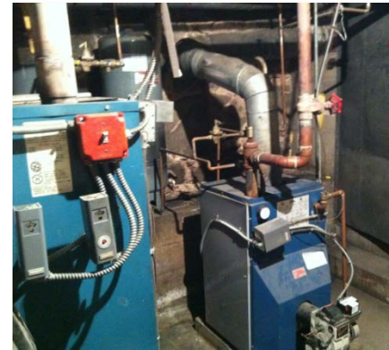
Figure 18: Hydronic Boiler Units
