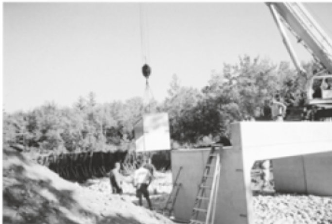
INSTALLING THE PRECAST CONCRETE
