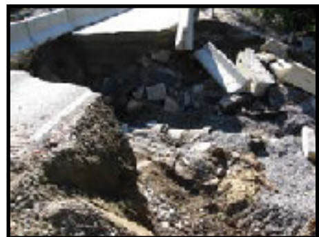
Depot Road culvert after Hurricane Hanna
