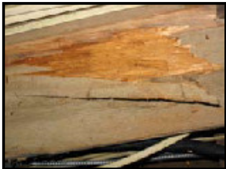
Close up of rotting support beam in the basement of Town Hall
