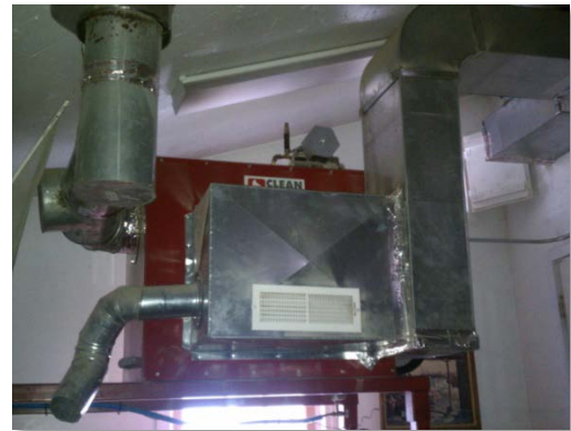
Figure 11: Waste Oil Furnace
