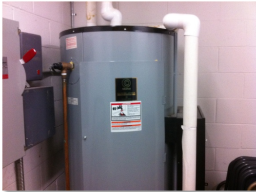
Figure 15: 119 Gallon Domestic Hot Water Tank
