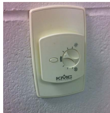
Figure 19: Cooling Controls in Computer Lab
