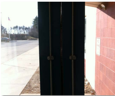
Figure 11: Gap in Door Parting (typ.)
