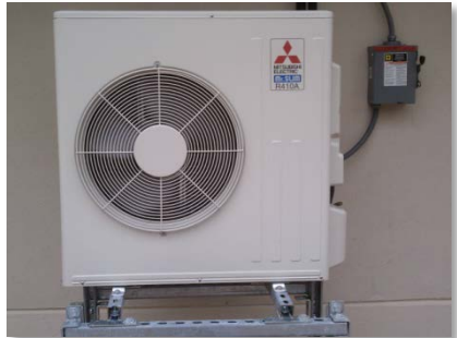
Figure 18: Mitsubishi® AC Unit Serving Computer Room
