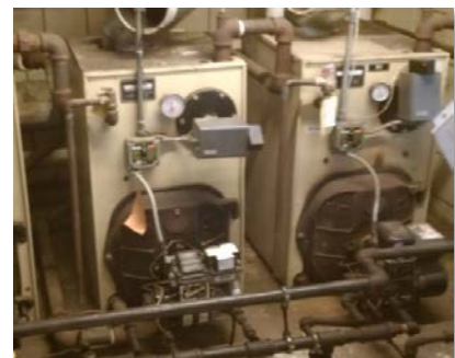
Figure 17: Weil-McLain® Oil-Fired Boilers
