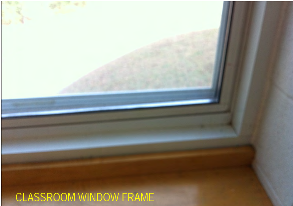
CLASSROOM WINDOW FRAME SHOWS THERMAL BREAK
