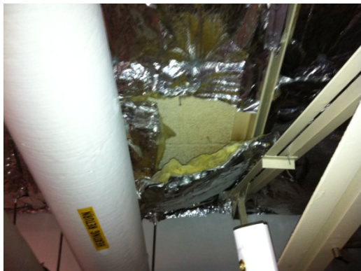
Figure 7: Ceiling Insulation on 1980 Roof
