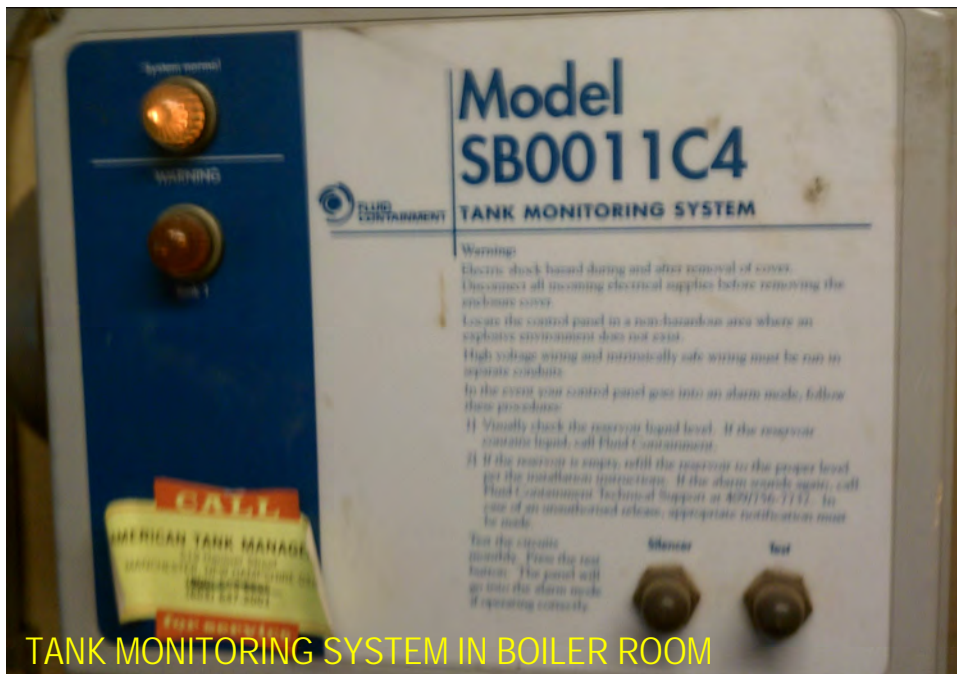
TANK SENSOR ALARM IN BOILER ROOM
