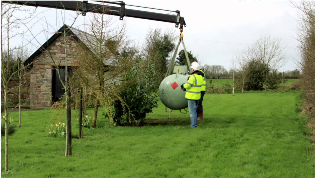
Installing an Underground Storage Tank
