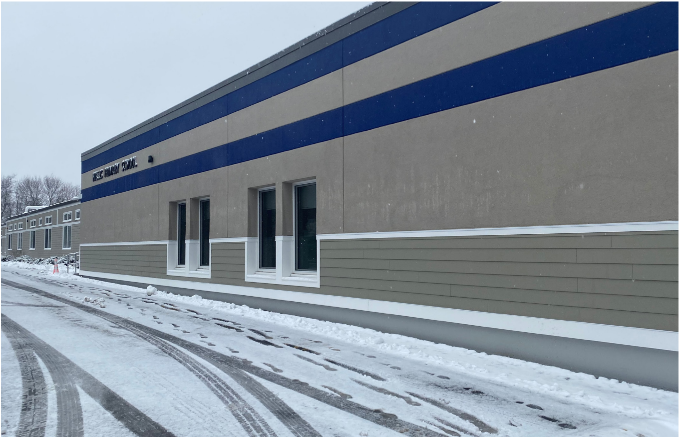
“Completion of the Summer 2022 Hollis Primary School cladding project”
